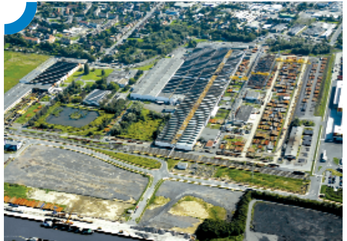
Salzgitter Mannesmann Line Pipe in Hamm
